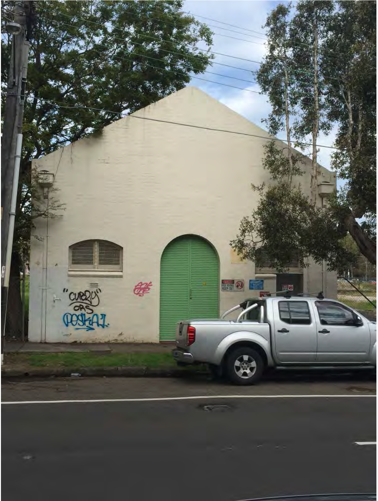
Figure 10: Ausgrid Heritage listed Sub Station – Young Street
