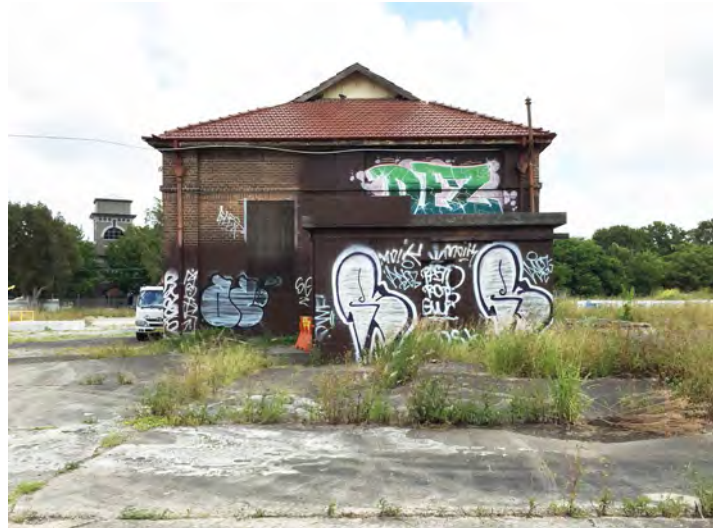
Figure 8 – Heritage listed Valve House, owned by Sydney Water (4)
